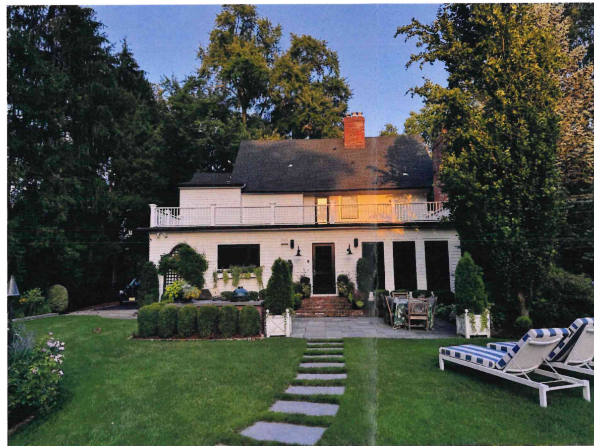
REAR OF HOUSE View to the East
